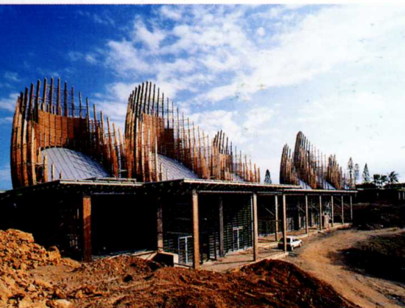
The enclave on its small peninsula permits the sea to be seen from the two main facades. The smaller one looks towards the interior of the island.
