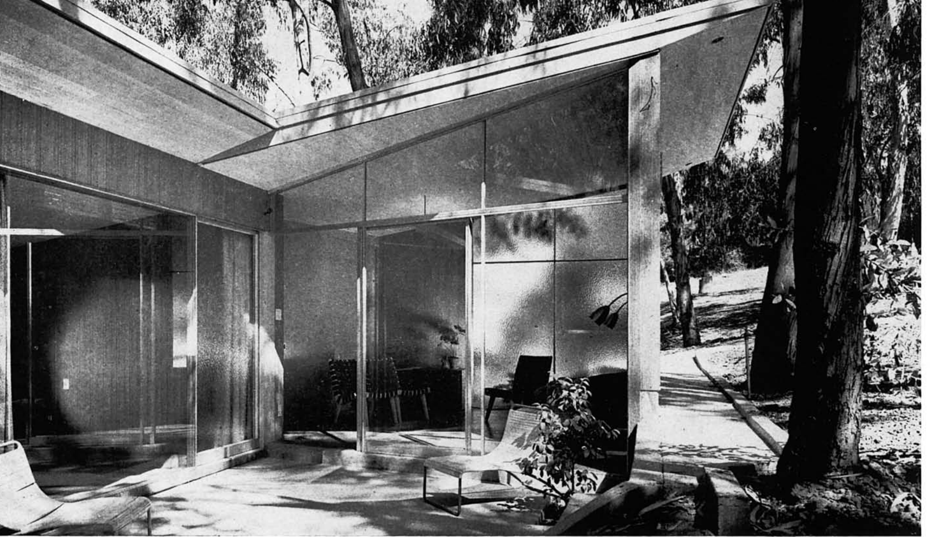
Above — The inward deviation of the studio wall gains a protecting corner roof overhang for the guest room sliding window.
