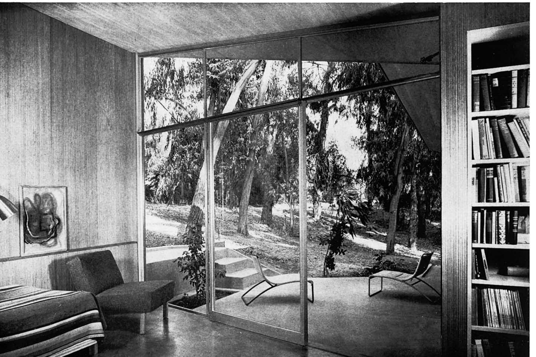
Below — A continuous floor slab and the entire glass wall merges the studio room with the terrace and surrounding landscape.
